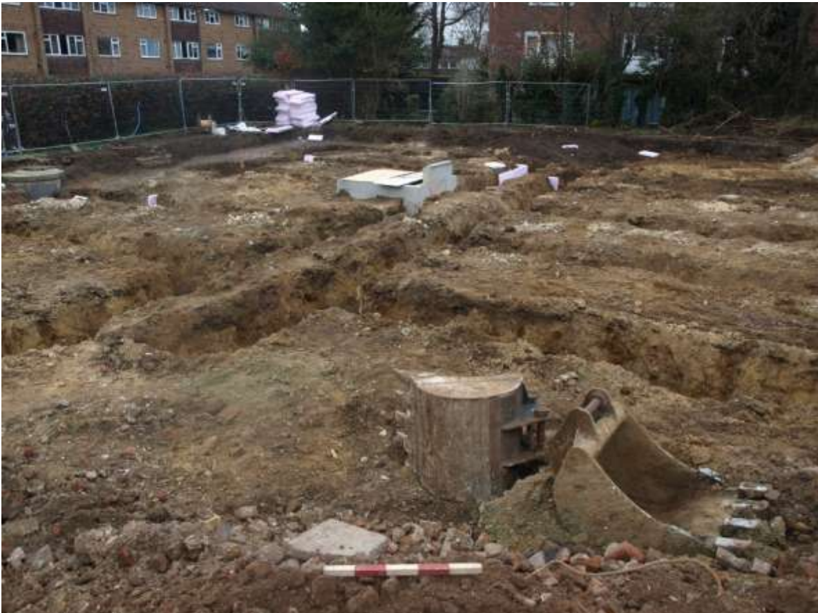
Plate 13: Foundation trenches and Plate 14 (below) overall view of foundation trenches
