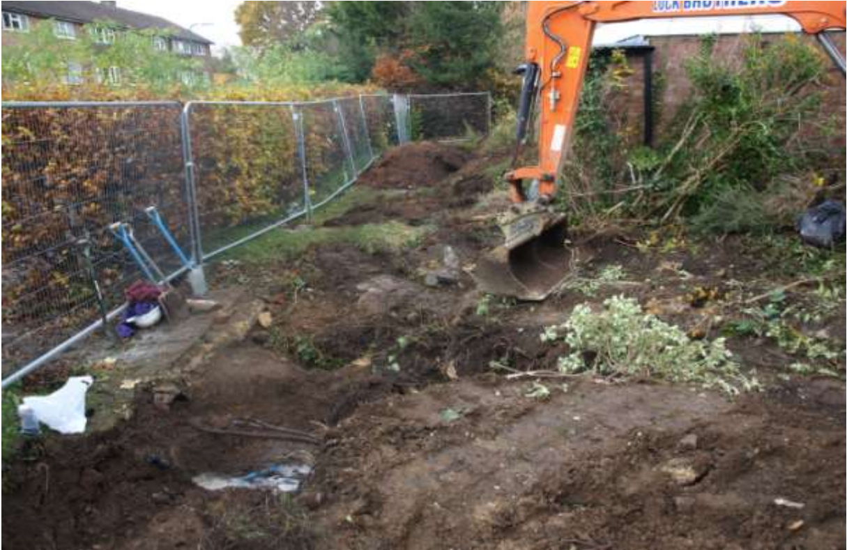
Plate 9: Showing eastern end of evaluation Trench 3, live water-main visible in foreground. Looking west, one and half-metre scales.
